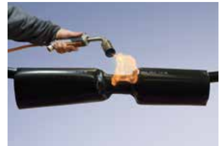
Apply the heat shrinkable tube
